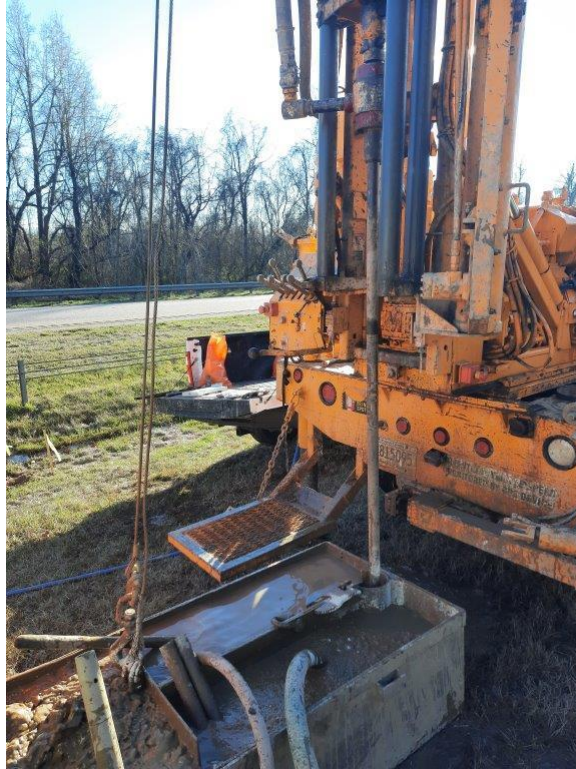
Drill rig on CO-4
