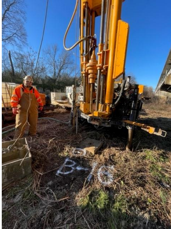
Drill rig on B-16
