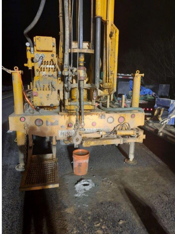
Drill rig on R-5
