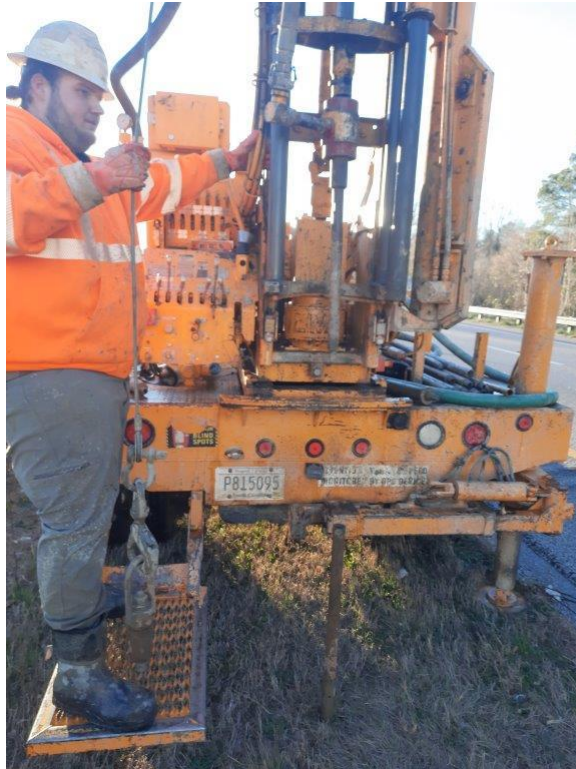
Drill rig on CO-3
