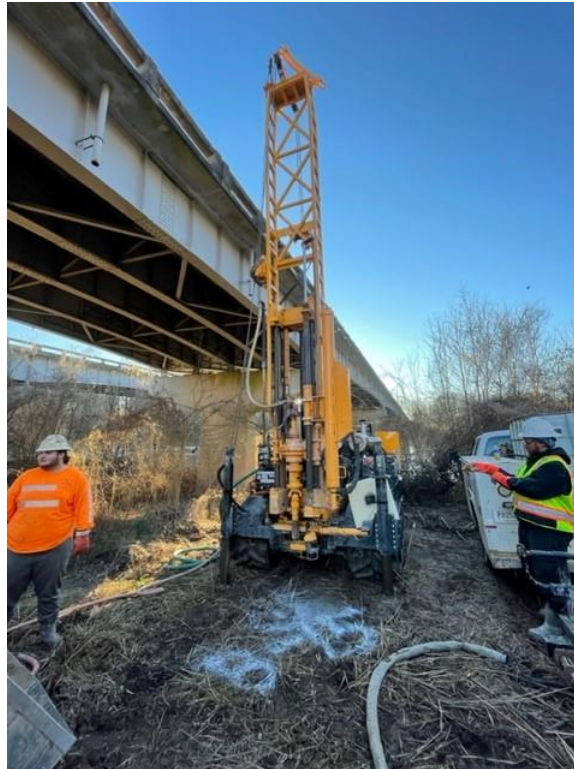
Drill rig on B-15
