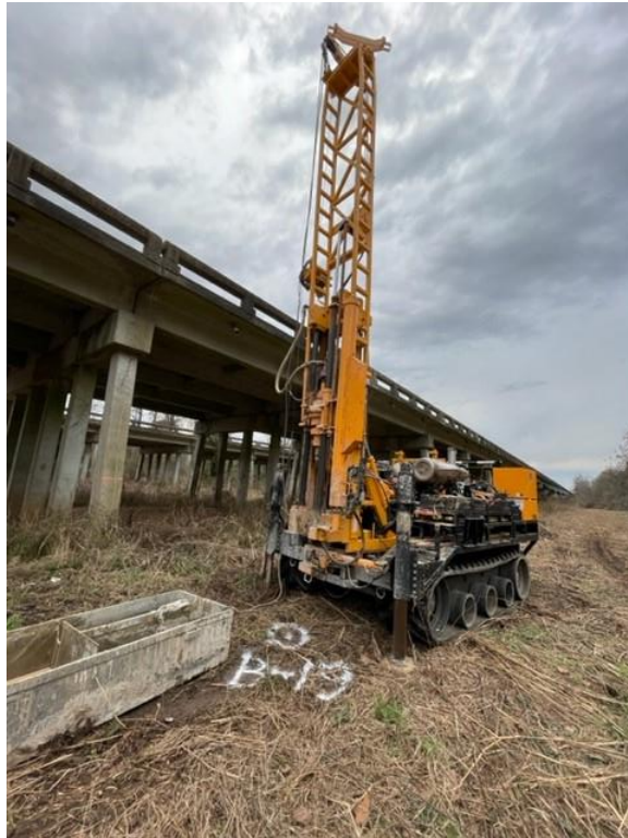
Drill rig on B-19
