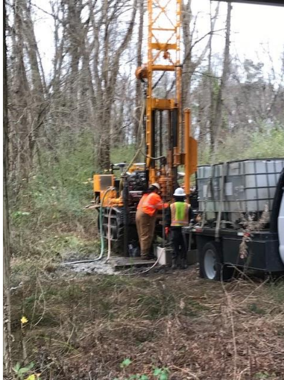
Drill rig on B-10
