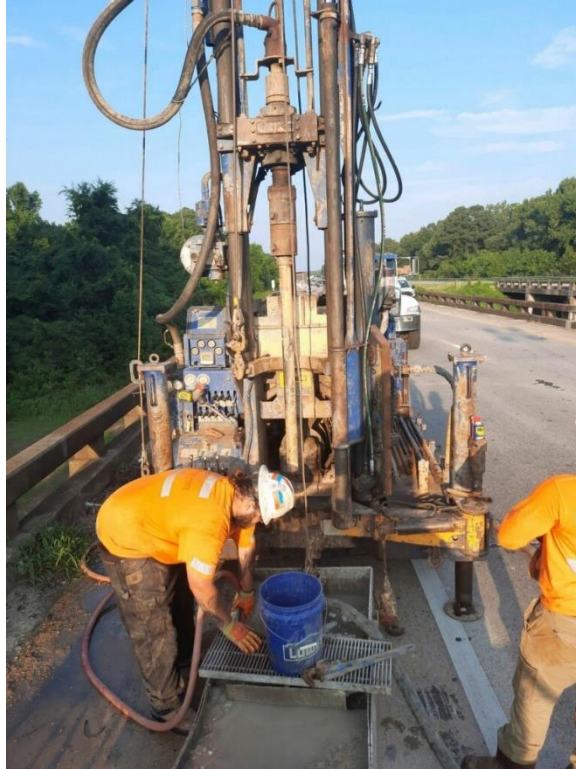
Drill rig on B-1
