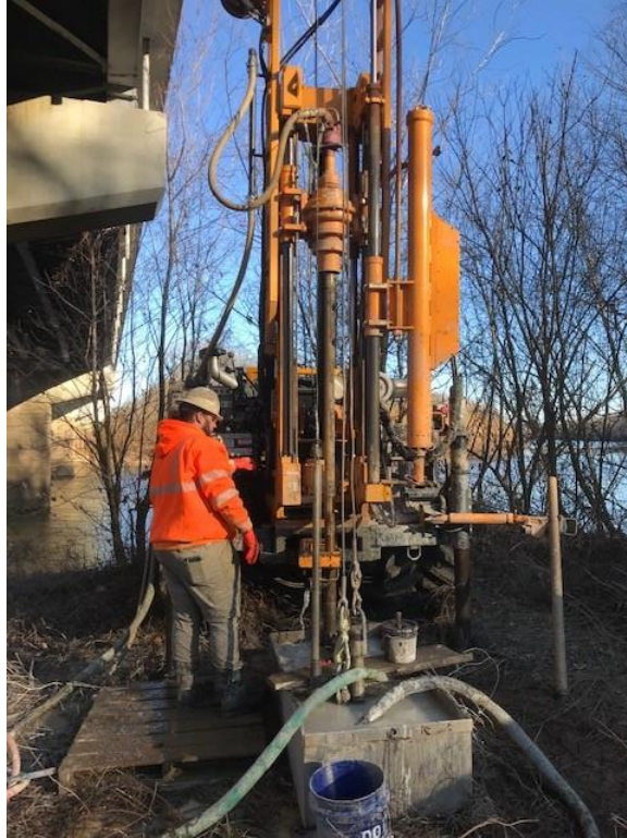
Drill rig on B-12
