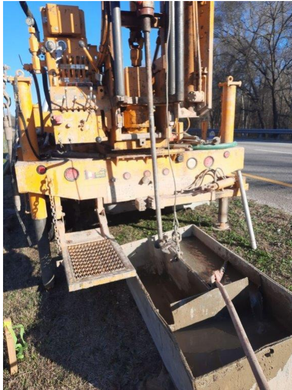
Drill rig on E-1
