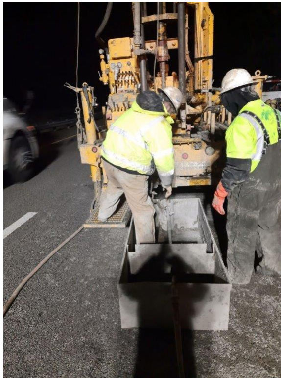
Drill rig on R-2
