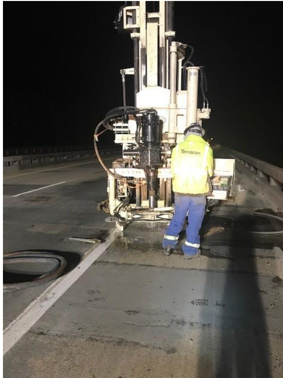
Drill rig on B-13
