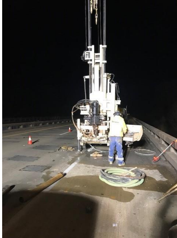
Drill rig on B-14
