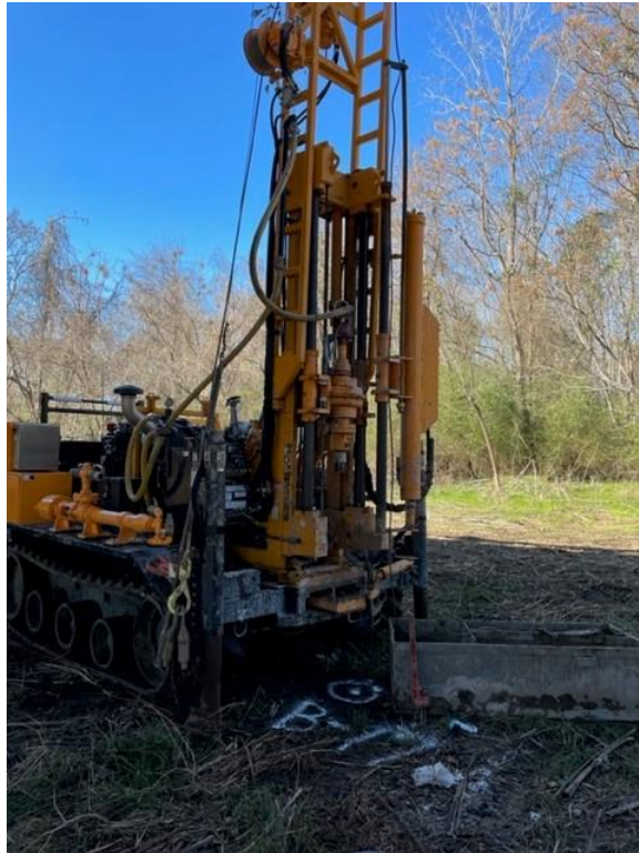
Drill rig on B-17
