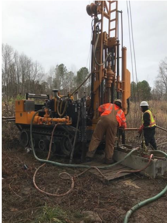
Drill rig on B-11
