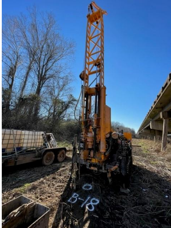
Drill rig on B-18
