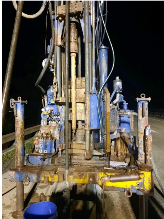
Drill rig on B-2
