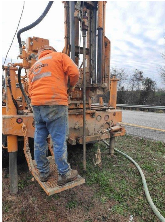
Drill rig on CO-1
