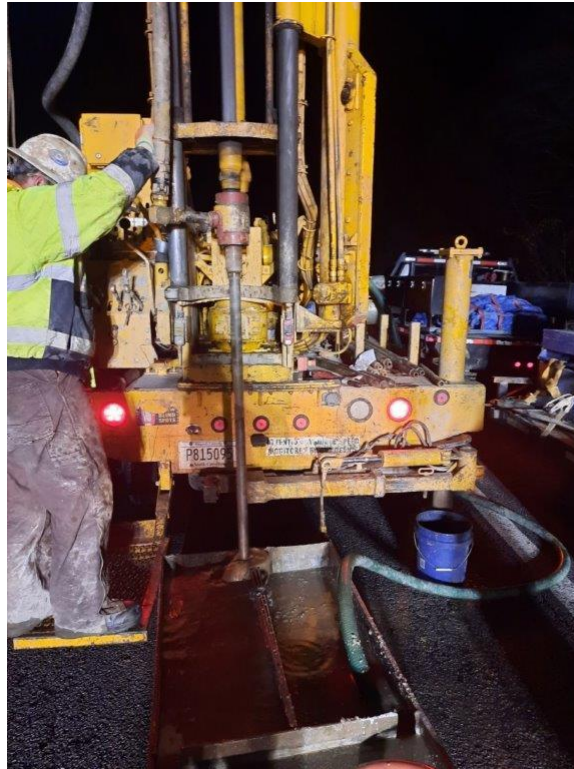
Drill rig on R-9
