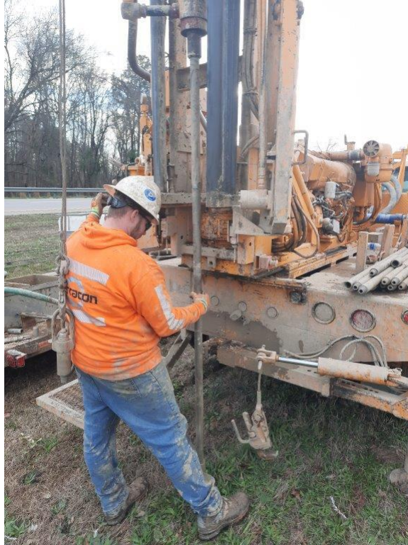
Drill rig on CO-2
